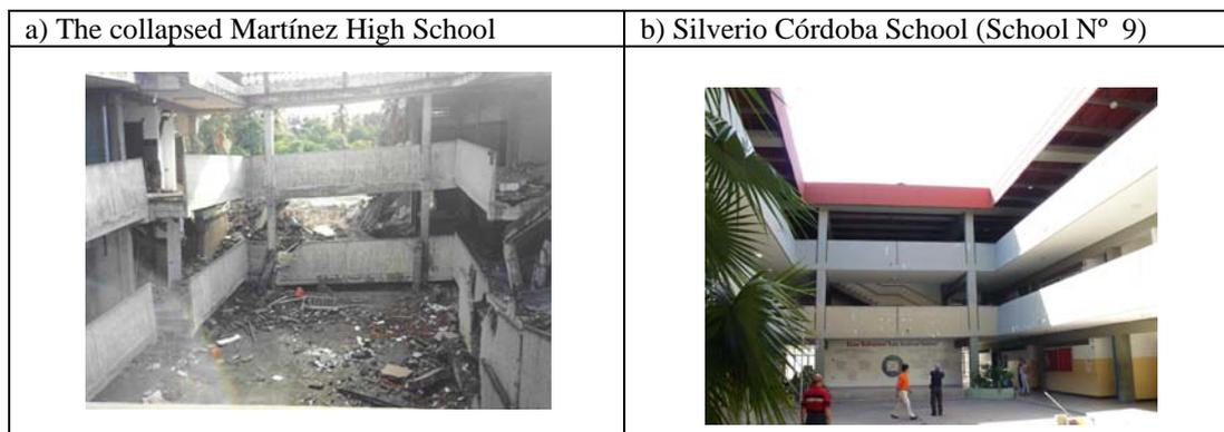
**Figure 2.** There are 334 school buildings of the Box-Type, similar to the collapsed buildings in the 1997 earthquake.
