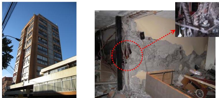
**Figure 1.1.** Damage of multi-story bearing wall without boundary columns at the 2010 Chile Earthquake
