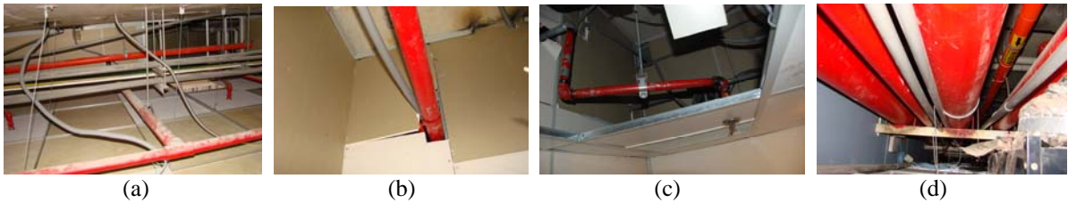
Figure 2.2. Investigation results of the sprinkler system damaged in 2010 Jia-sen earthquake: (a) bed area (b) from shower room to bed area, (c) entrance, and (d) corridor
