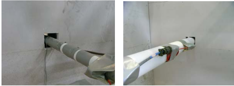
Figure 3.5. Clear spacing between the partition board and the branch
