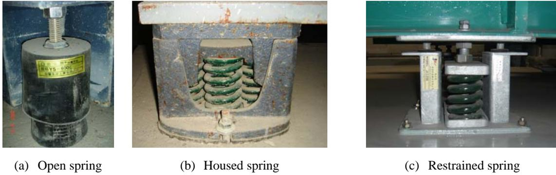
**Figure 1.2.** Commonly used spring isolator types in Taiwan
