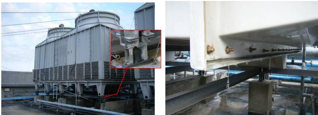
**Figure 1.1.** Leakage damage of a spring isolated cooling tower at the roof level after Hwa-Lien earthquake
