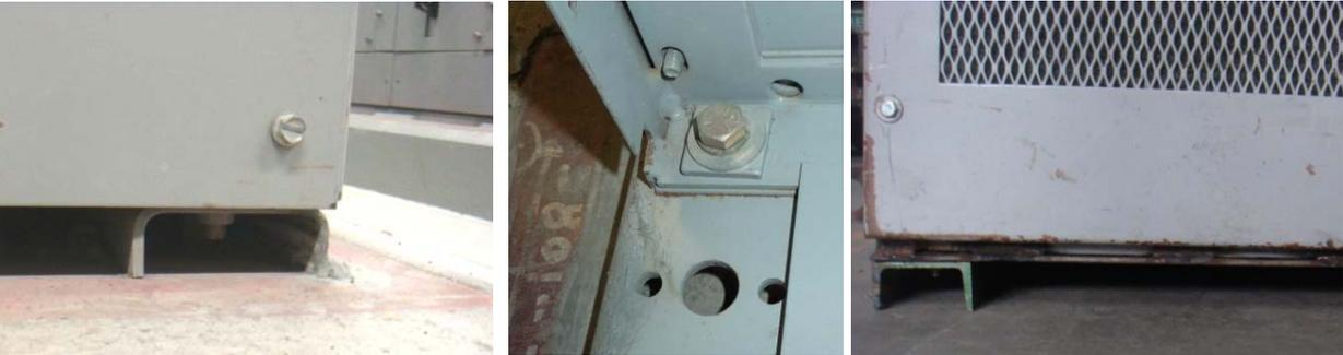
Figure 2.2. Anchorage of Test specimen
