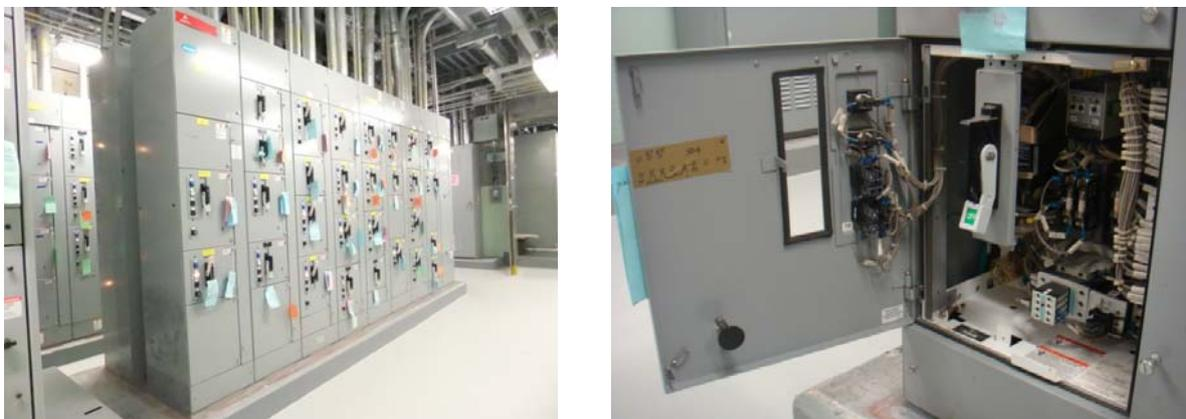
**Figure 1.2.** MCC cabinets belonging to RHR C system in NPP4
