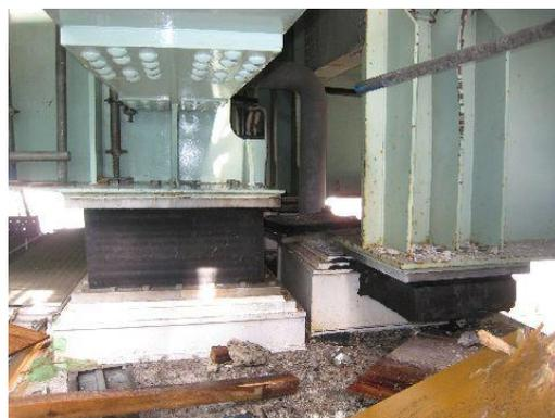
**Photo 1.1.** Damage of the bridge rubber bearing
