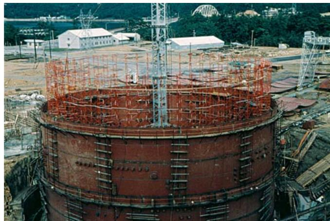
**Figure 6.** The base of the steel structure at the early phases of construction of the Fukushima Daiichi NPP, by courtesy Watabe (1970).
