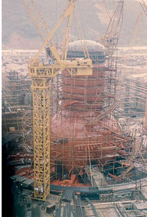
**Figure 7.** The containment vessel of the Fukushima Daiichi NPP almost finished, by courtesy Watabe (1970).
