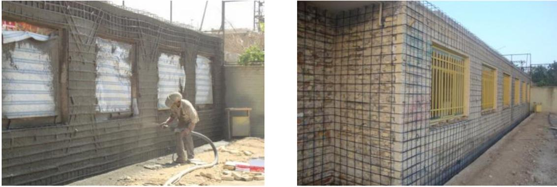
**Figure5:** Samples of retrofitted school buildings with peripheral shotcrete
