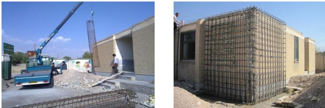
**Figure3:** Samples of retrofitted school buildings with shear walls
