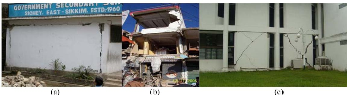
**Figure 6.** Failure of infill masonry walls: (a) Out-of-plane tilting of masonry infill wall (India); (b) Out-of-plane failure of infill walls in Pakistan (Bothara et al., 2008); (c) Diagonal failure of infill walls separated from columns, Indonesia
