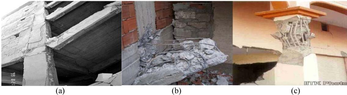
**Figure 7.** Failure due to lack of ductile detailing: (a) non-ductile details for beam-column joints, Bingo Turkey (Sezen et al., 2003); (b) poor detailing, India (Jain & Murthy, 2001); (c) collapsed column (note the absence of stirrups in a column length larger than 700 mm), Pakistan, 2008
