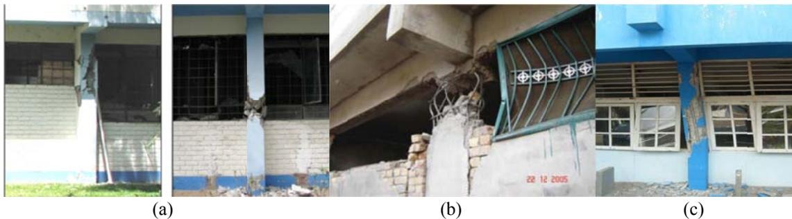
**Figure 2.** Short-column mechanism; (a) Turkey (Dogangun, 2004); (b) Pakistan (Bothara *et al.*, 2008); (c) Indonesia (Ghobarah *et al.*, 2006)
