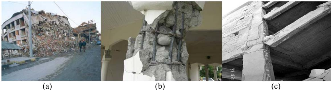
**Figure 8.** Failure in buildings with low materials quality: (a) poor quality of concrete, Turkey (Arslan & Korkmaz, 2008); (b) segregation of concrete and large pebbles/cobbles in the concrete, 90° hooks and wide spacing of stirrups, Indonesia, 2010; (c) damage due to poor material quality in beam-column connection, Turkey (Sezen, 2003)
