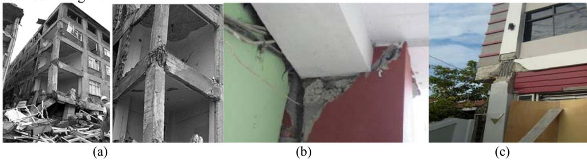
**Figure 4.** Failure of beam-column joints: (a) Building collapse due to failure of beam-column joints, Turkey (Sezen et al., 2003); (b) Poor seismic detailing of RC frame members and beam-column joints, India (Murthy, 2001); (c) No stirrups in beam-column joint, Indonesia (Bothara et al., 2010)
