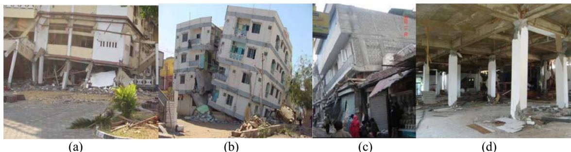
**Figure 3.** Soft-storey failure mechanisms: (a) Indonesia (Bothara *et al.*, 2010); (b) Bhuj Earthquake, India (Murthy, 2001); (c) Pakistan; (d) Plastic hinging of columns of an open bottom storey, Indonesia (Bothara *et al.*, 2010)
