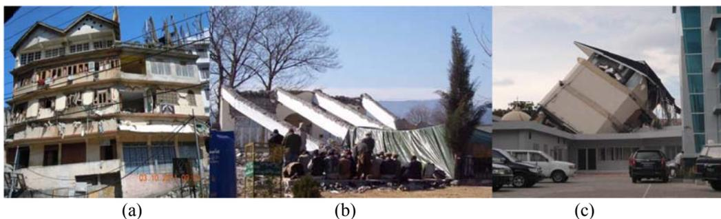
**Figure 5.** Failure due to strong-beam weak-column mechanism: (a) Pan-caking failure of school-cum-residential building at Chungthang, India (Murthy, 2001); (b) Strong-beams weak-joint and columns, Pakistan; (c) Building collapse due to column failure, Indonesia (Bothara et al., 2010)
