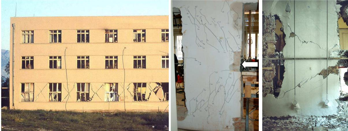
**Figure 1.** Typical earthquake damage of masonry building and in-situ shear test
