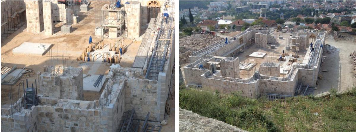
**Figure 4.9.** Construction of the church up to the level of first horizontal ties
