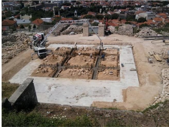
**Figure 1.2.** Newly designed RC foundation in the course of construction
