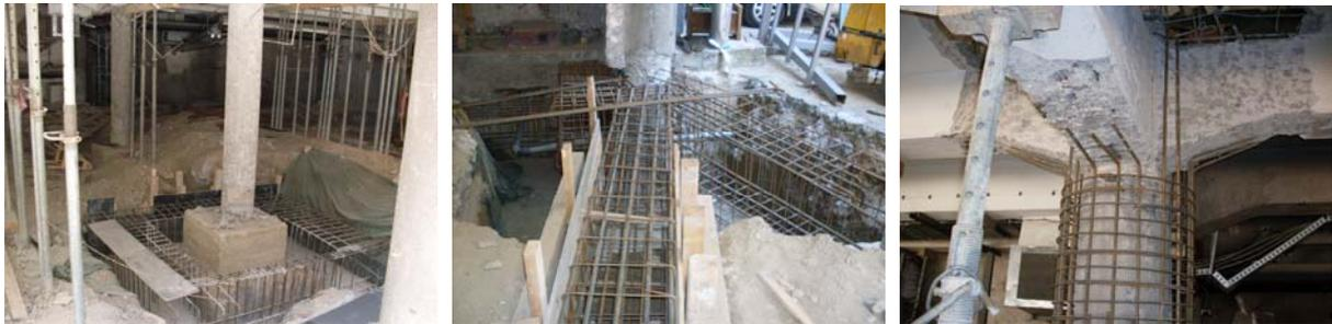
**Figure 5.1.** Strengthening of a characteristic column with a plastic hinge, Unit 3
