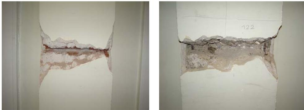
**Figure 2.2.** Research boreholes in corridor pilasters (left – brick, right – RC column)
