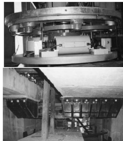
**Figure 5.** Passive Energy Damping Devices Incorporated in West Bolu Viaducts (GEER 1999 and Roussis et al. 2003)
