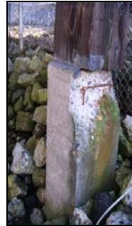
**Figure 16.** (a) Side view of pier and its foundation (b) Close-up of a wooden post on spalled concrete post.
