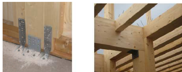
Figure 6. An example of ground connection and wood to wood connections
