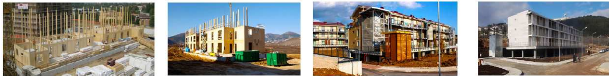
Figure 3. Different assembling steps of a 3-storey Dolomiti Plus building in Italy located in L'Aquila and the building completed for -Progetto C.A.S.E.- (photo-credit ILLE Prefabbricati s.p.a)
