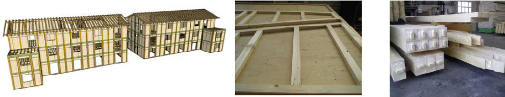
Figure 2. Design model of the main structures; panel's frame on the production's bench and ready main wooden structures
