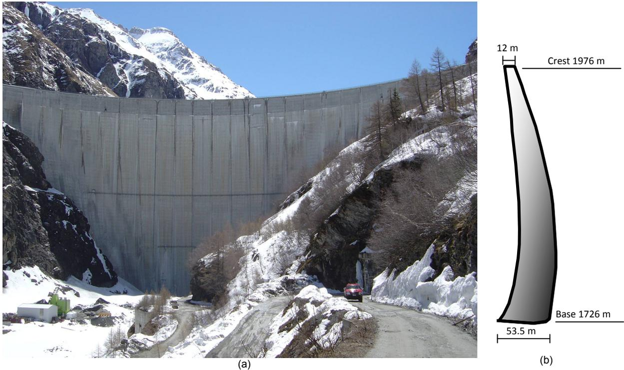
**Figure 1.** Mauvoisin Dam, Switzerland: (a) view from the downstream; and (b) cross-section of crown cantilever
