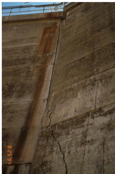
**Figure 12.** Joint opened and cracks occurred in the thrust block of Pacoima Dam during the Northridge earthquake
