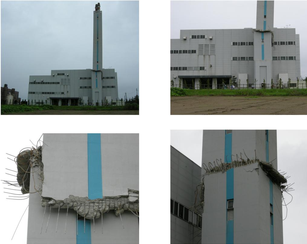
**Figure 1.** Damage of the chimney
