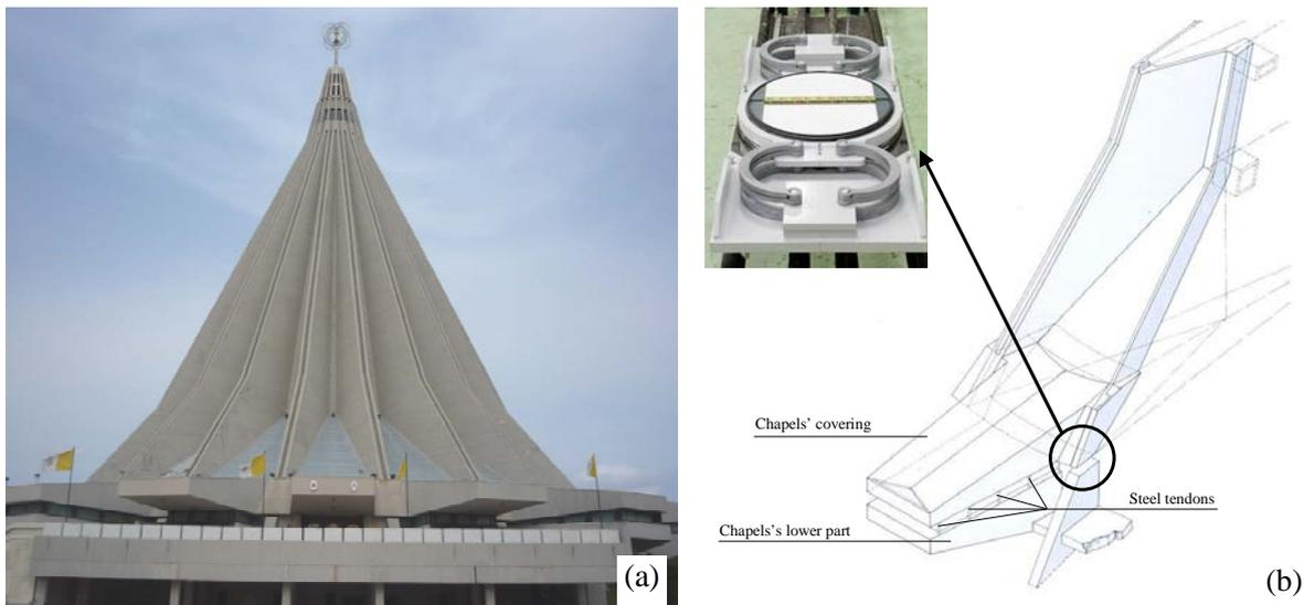
**Figure 1.1.** (a) View of the Sanctuary, (b) axonometric view of one chapel and the base ring
