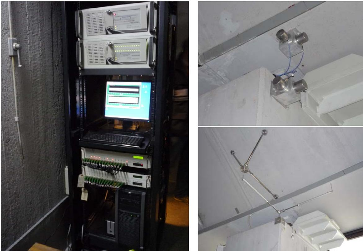
**Figure 1.3.** Acquisition/processing/storage system and sensors for the monitoring of the Sanctuary
