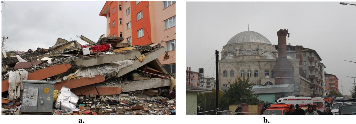
**Figure 11.** Extent of structural damage along Vanyolu Street, Ercis: a. totally collapsed building due to soft story mechanism; b. collapsed minaret of Van Yolu Mosque (GIT-EQ, 2011)
