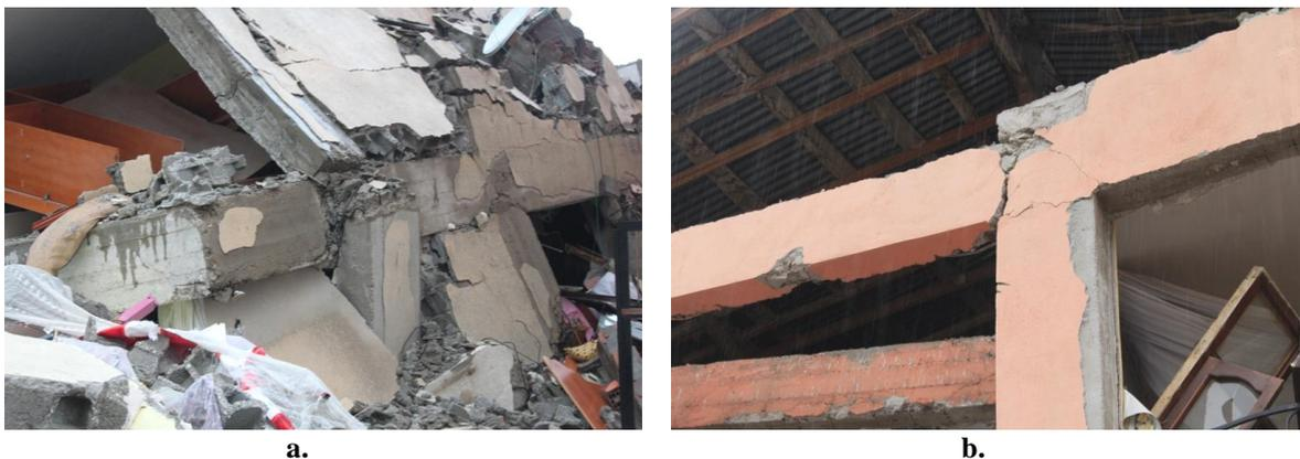
**Figure 12.** Beam-column joint failures in Ercis: a. failure in a beam-column joint due to inadequate confinement; b. brittle failure in a beam-column joint (GIT-EQ, 2011)
