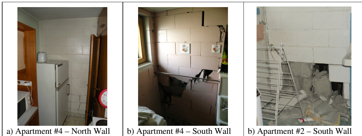
Figure 6. Damage to Interior Walls – East End
