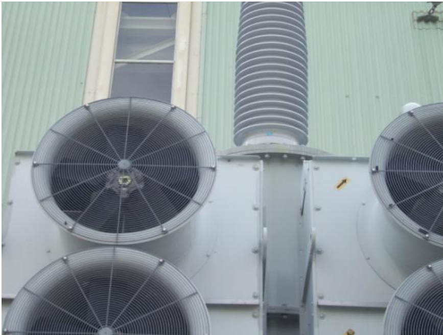
Figure 5. Transformer's bushing and the flange
