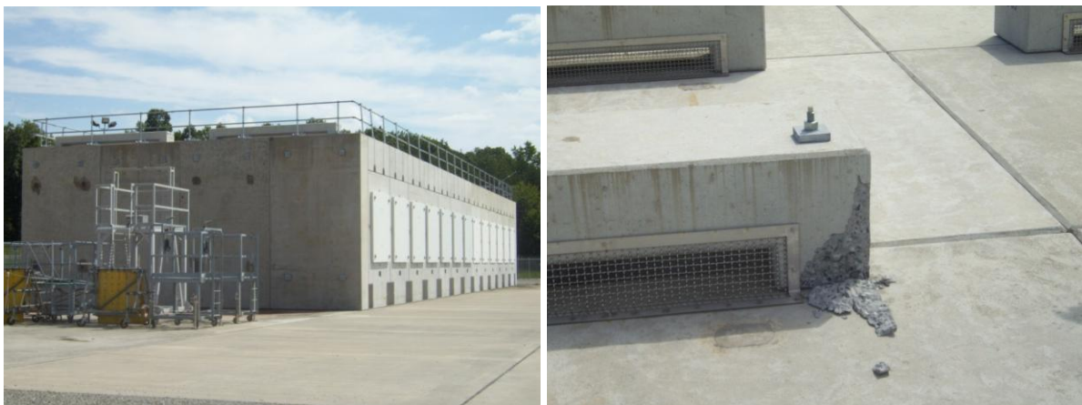
Figure 6. TransNuclear casks at the NANPS (left) and some of the casks were moved as far as 11.4 cm (right).
