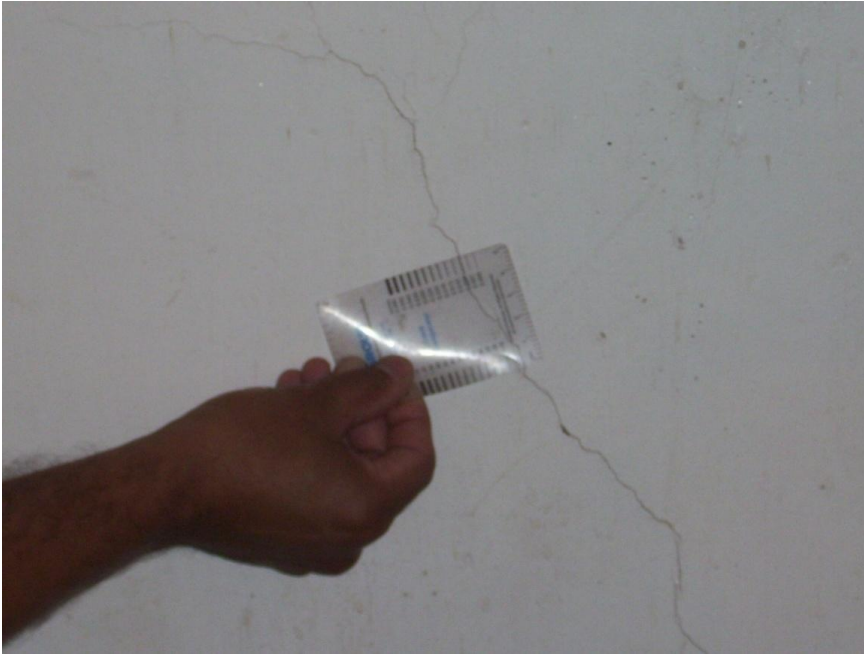
Figure 2. Inclined crack on the internal wall of turbine building. The width of the crack is about 0.25 mm
