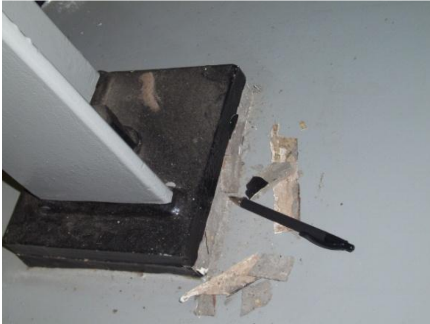
Figure 4. Spalling at an anchored Phase Separator tank base.
