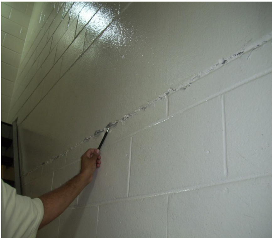
Figure 3. Horizontal cracks developed from construction joints between lifts in the Auxiliary building.
