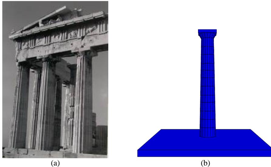
**Figure 2.** (a) View of the SE corner of the Parthenon. Behind the columns of the east façade the SE column of the Pronaos can be seen; (b) Numerical model of the column used in the analyses.
