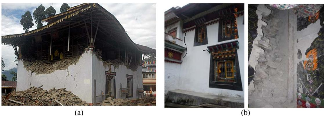
**Figure 3.1.** Common damages observed (a) Partial collapse of wall of Ringhem Choling monastery due to forces imposed by the roof deflection and (b) Shear cracks and delaminated wall painting at Samten Choling monastery.
