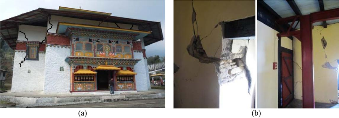
**Figure 3.3.** (a) Cracks on the exterior wall of Labrang monastery and (b) Exposed stone laminates during the recent damage and steel columns and joists used in the retrofit
