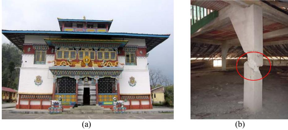
**Figure 3.4.** (a) Phodong monastery, interior RC frame with exterior stone masonry wall and (b) Damaged column due to short-column effect induced by the presence of deep haunches at beam-column junctions.
