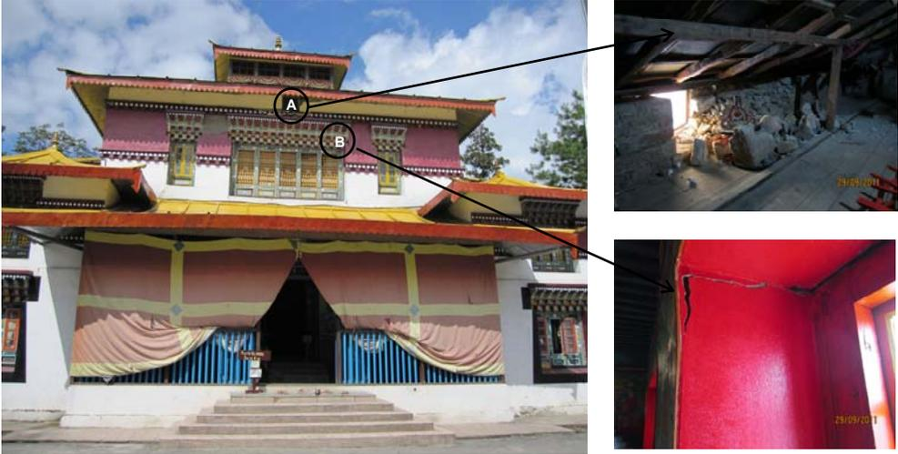
**Figure 3.2.** Damages observed on the front wall of third storey at Enchey monastery
