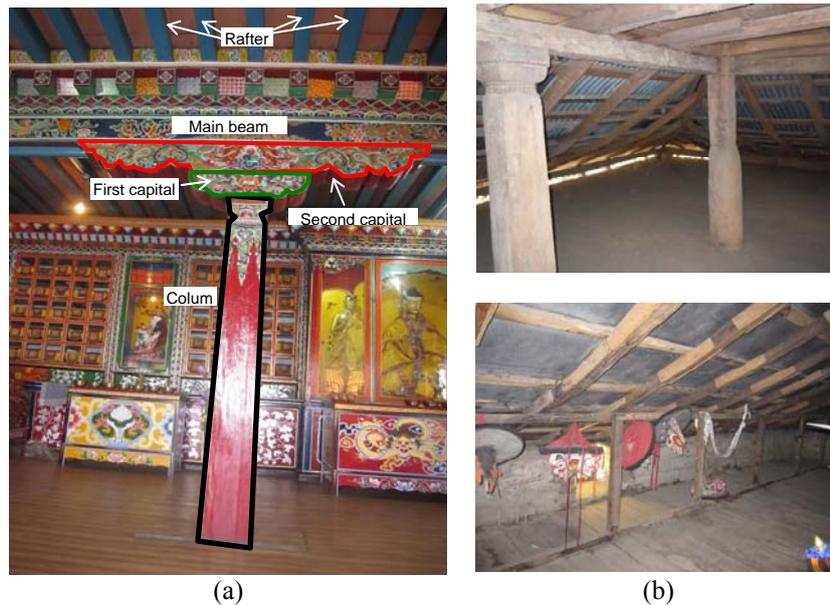
**Figure 2.2.** Details of (a) wooden timber frame and floor diaphragm supported on rafters and (b) hipped roof construction.
