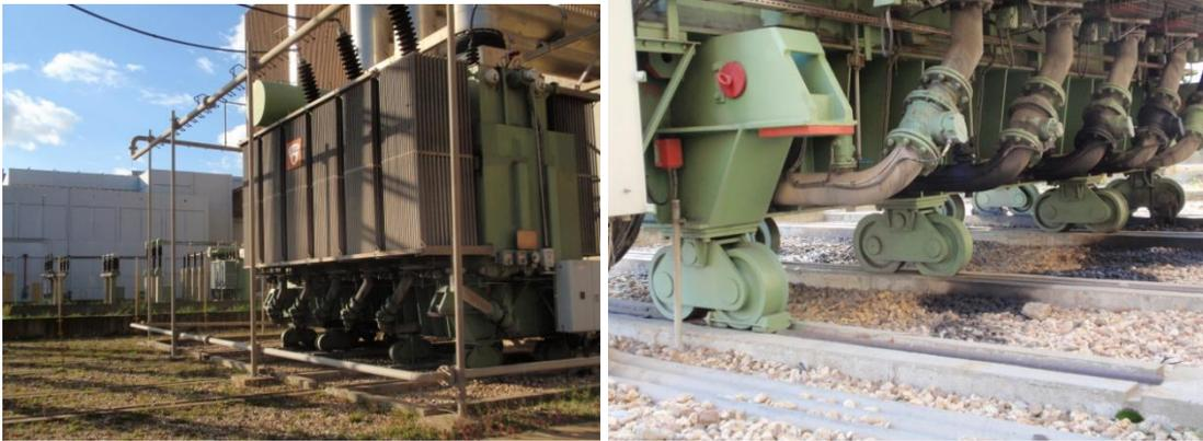
**Figure 6** - Power transformer supported on wheels
