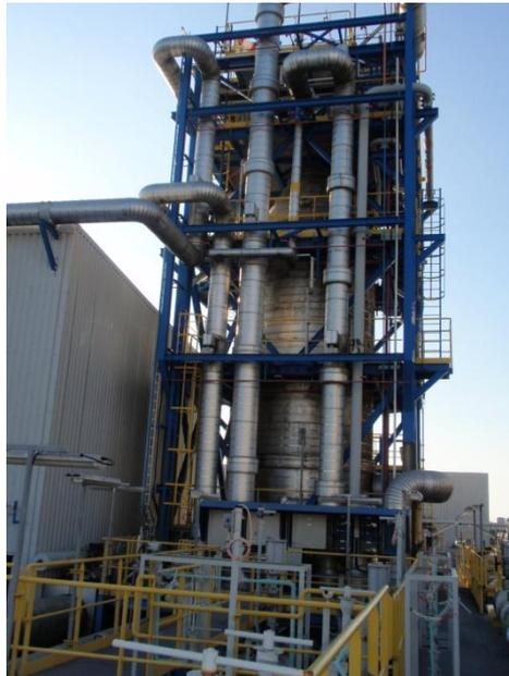
**Figure 4** - Steel structure braced for horizontal actions (in blue)
