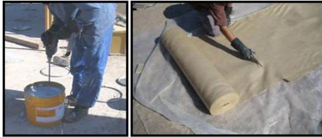
**Figure 14.** Mixing the two-component adhesive with a mixer (left) and cutting the jute mat to reinforce the walls
