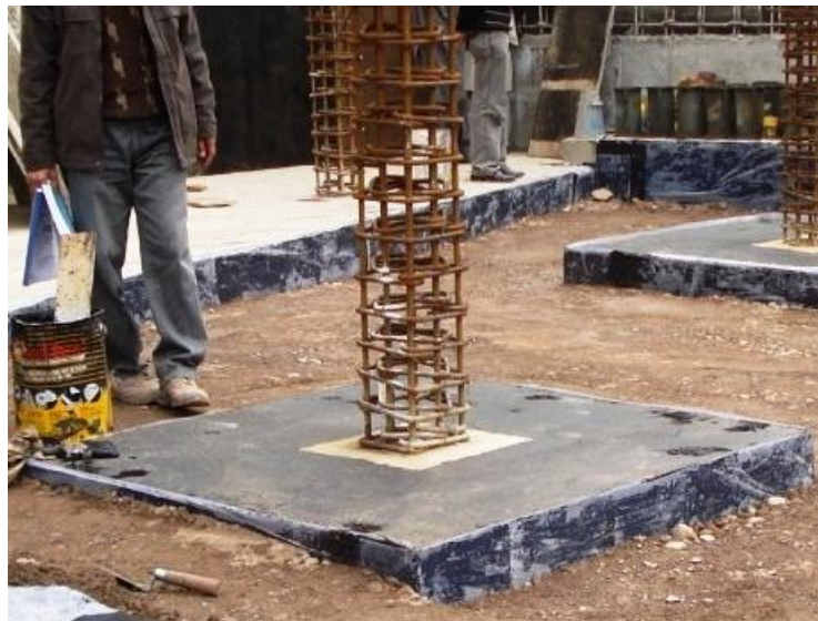
Figure 3.4. Column rebar cage construction photo
