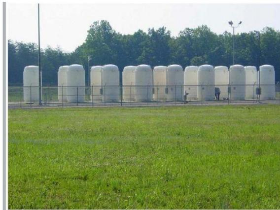
**Figure 3.** Dry casks placed vertically in robust above-ground concrete at North Anna nuclear power plant site (Close-up view) [10]
