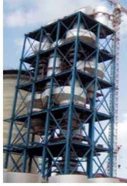
Figure 1.1 Picture of the braced steel frame structure
