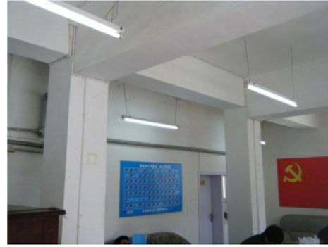
**Figure 2.1.** Inner frame-supported masonry structure
