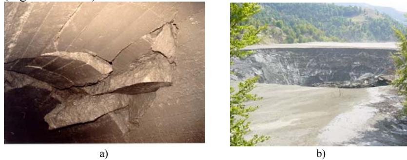
**Figure 2.** Partial collapse of diversion tunnel and occurrence of sinkhole for the waste surface area of tailing dam 2
