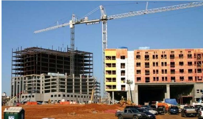
**Figure 1.1.** Examples of concrete/steel and concrete/timber mixed construction with a change in construction material over the height in North Carolina (image courtesy of the Independent Weekly)
