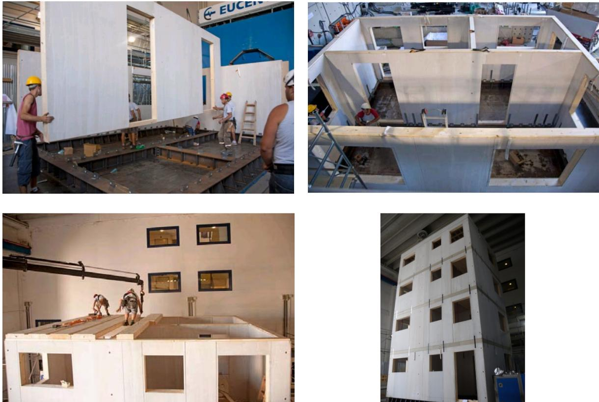
**Figure 2.1.** Construction phases of the tested structure
