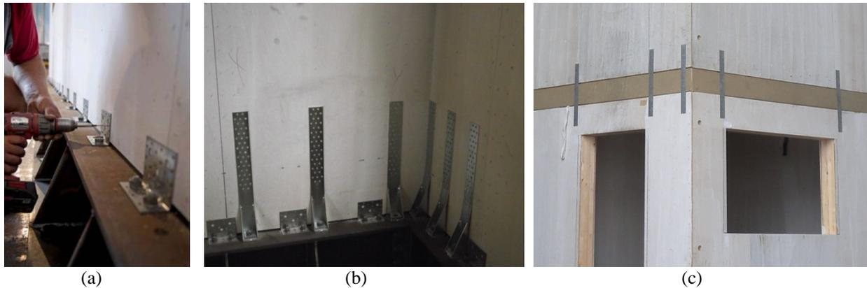
**Figure 2.2** Steel connectors: (a) brackets; (b) hold-down; (c) tie-down
