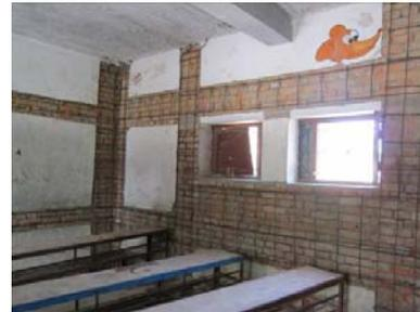
**Figure 6:** RCC splints and bands on interior walls
