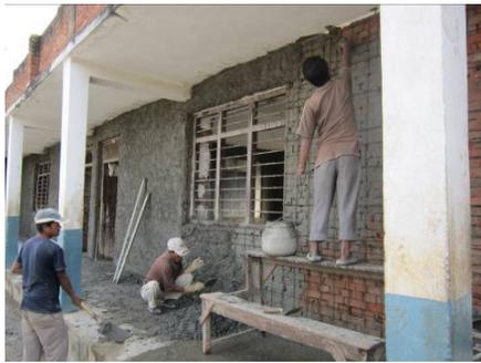
**Figure 9.** Micro-concreting grouting
