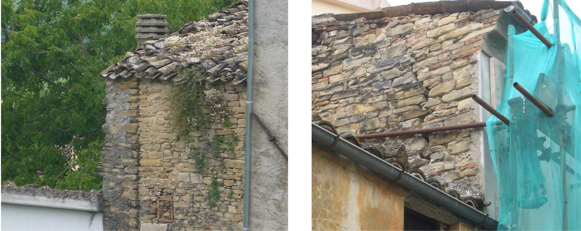
**Figure 4.2.** Global out-of-plane mechanisms
