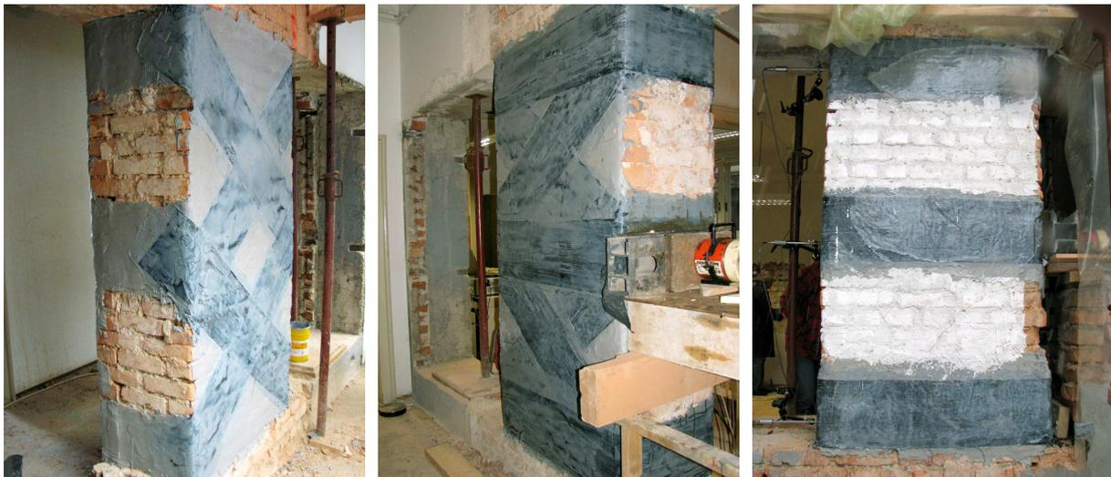
**Figure 8.** The application of carbon fiber fabric in epoxy resin: specimen H1w after placing the inclined strips on one side (left), complete specimen H1w with inclined strips and horizontal strips, equally on both sides (middle) and the outer side of specimen H2w only with horizontal strips (right)
