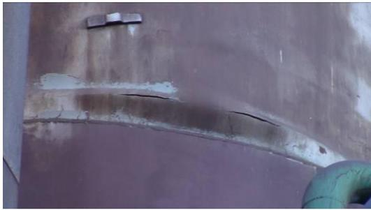
(c) Buckling of chimney wall
