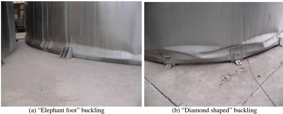
**Figure 7:** Tank wall damage
