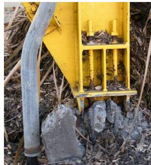
**Figure 5:** Stretching of anchor rods and pedestal failure
