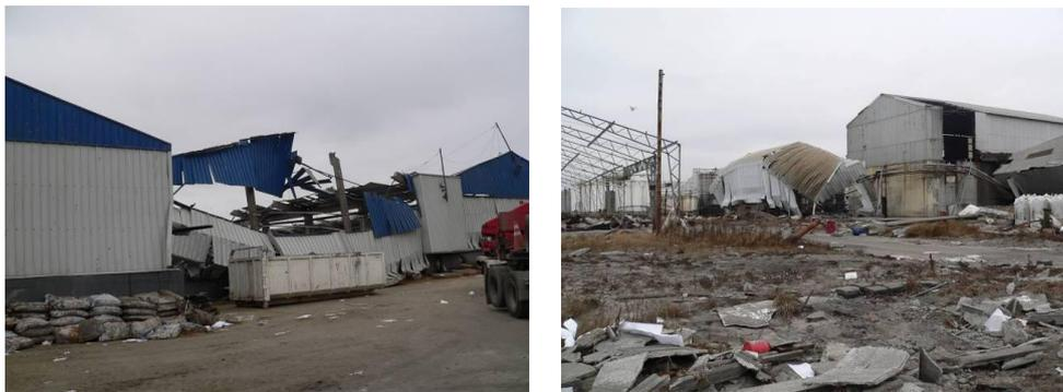
**Figure 8:** Damage on fish processing plants in Talcahuano.
