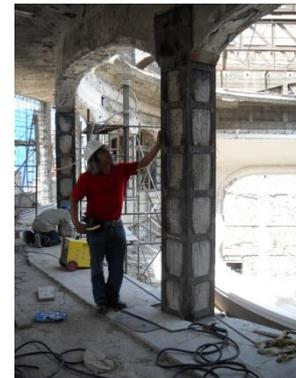
Figure 21. View of column after retrofitting.
