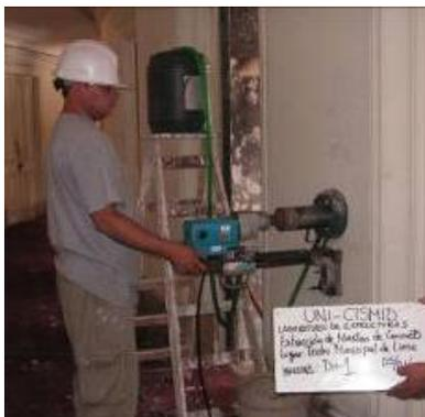
Figure 13. Concrete sample from concrete Wall in 1<sup>st</sup> floor.
