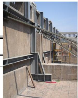
**Figure 31.** View of the retrofitted wall.
