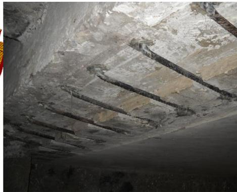
**Figure 28.** Union of some slabs through anchors.
