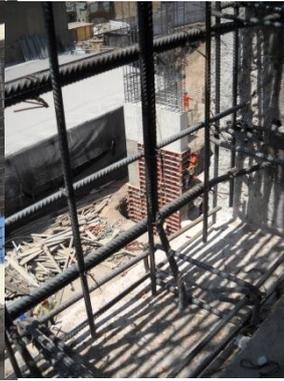
**Figure 25.** Anchorage of steel bars in concrete frame elements.
