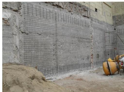
Figure 23. Retrofitting external wall view.
