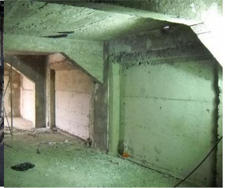
**Figure 26.** New concrete infill shear walls in the structure.
