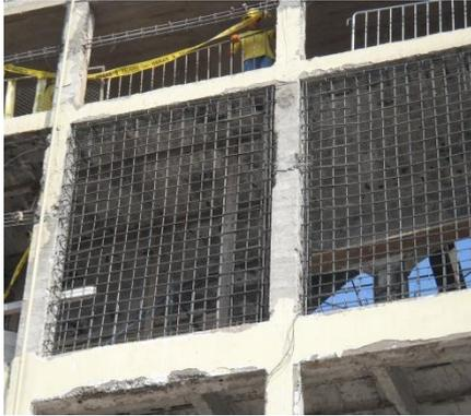
**Figure 24.** Infill shear wall Steel mesh in between frame elements.
