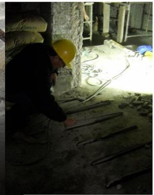
**Figure 29.** Union of some slabs through anchors.
