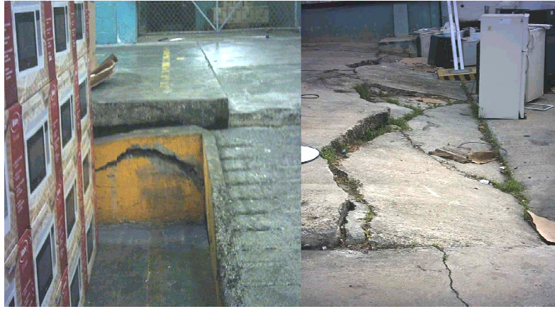
Figure 3. Pavements Elevations and Cracking in Pavements Slabs.
