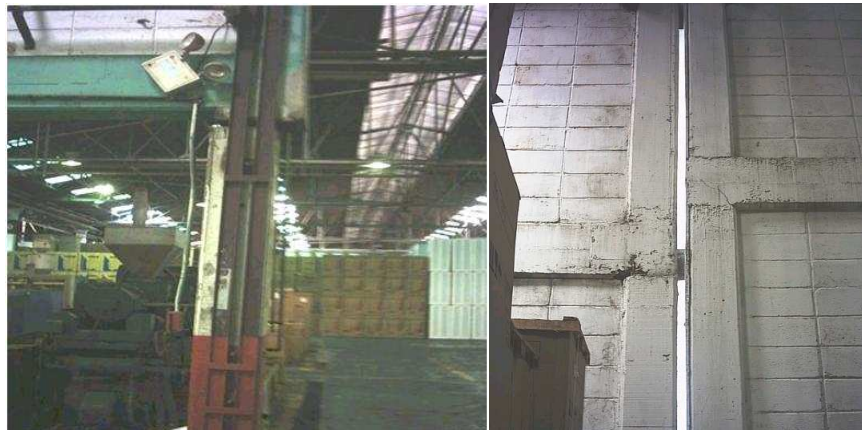
Figure 2. Excessive Columns Deformations and Differential Settlements in Structures.
