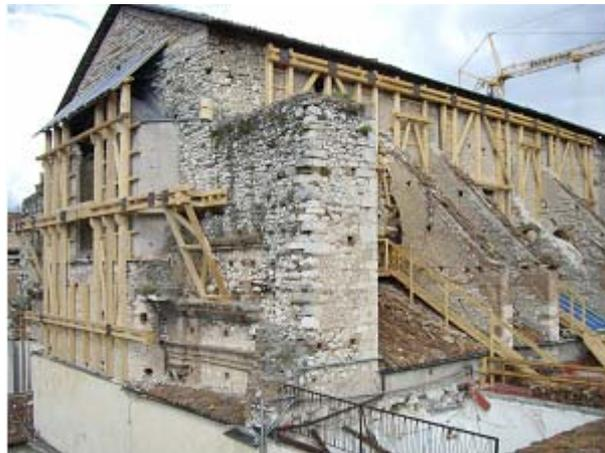
**Figure 8.** Santa Margherita Church, L'Aquila (AQ). Tightening of the apse wall and main barrel vaults.
