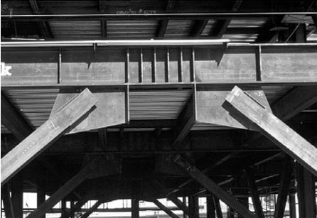
**Figure 2.7** Example of eccentrically braced frame
