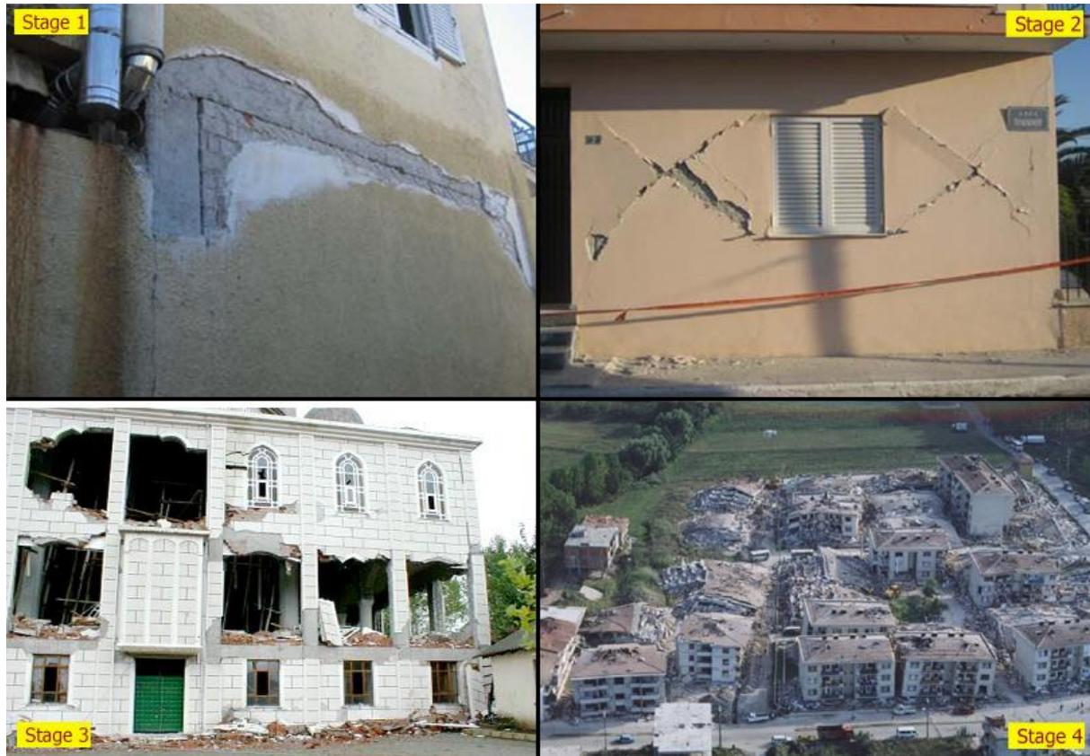
**Figure 1.** Stages of infill wall failure on RC structures (from small cracks up till total collapse)
