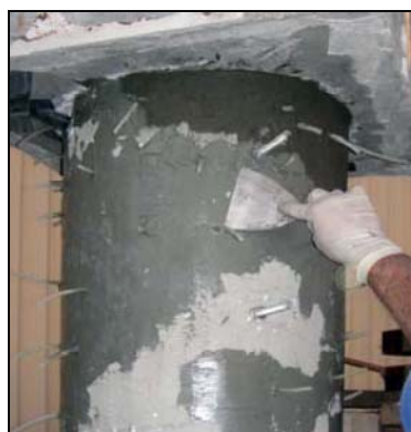
(a) Cap sealing and surface repair
